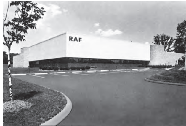
U.S. manufacturing and plating facility
